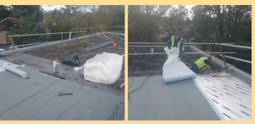
Corstophine Roofing and building have recently started on the roofing work at our Woodthorpe development at Redford Road. This significant investment will see all three major roofs stripped, reinsulated and recovered with modern, long lasting roofing materials, along with slate repairs to the old building.
